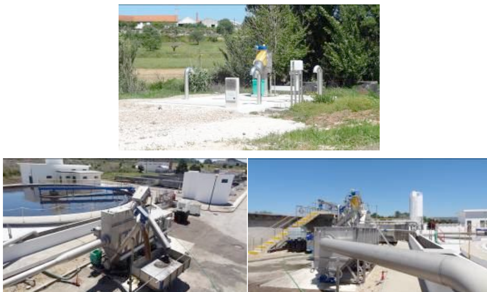
Figure 2.9. Pretreatment of domestic effluent (compact unit with degreaser)
