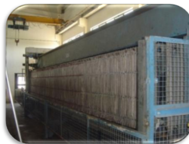
Figure 2.18. Filter press for sludge dewatering
