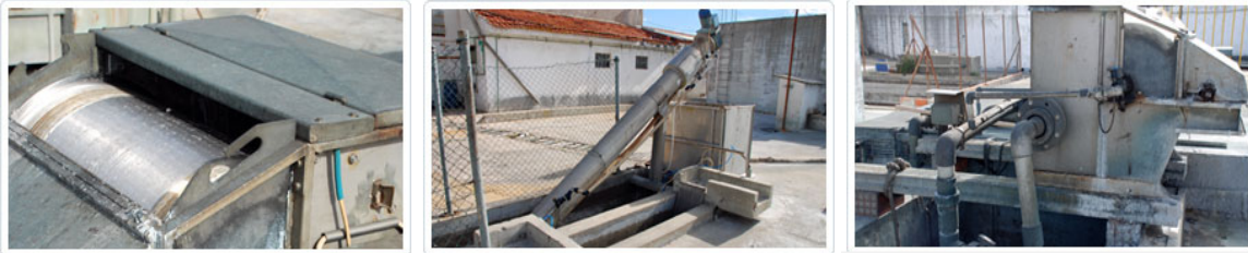
Figure 2.6. Fixed grids and rotary screens
