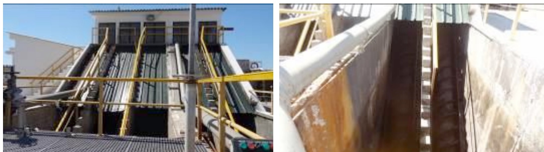
Figure 2.10. Archimedes screws and electric pump groups
